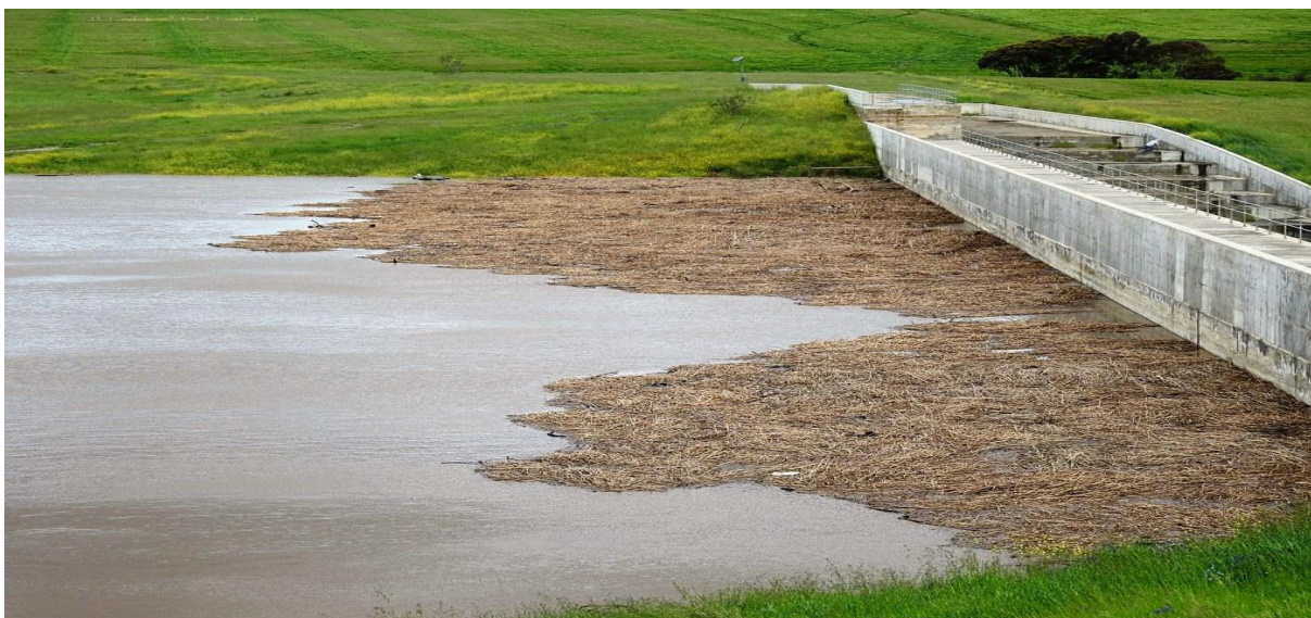
Image 5: Flood mitigation dam
